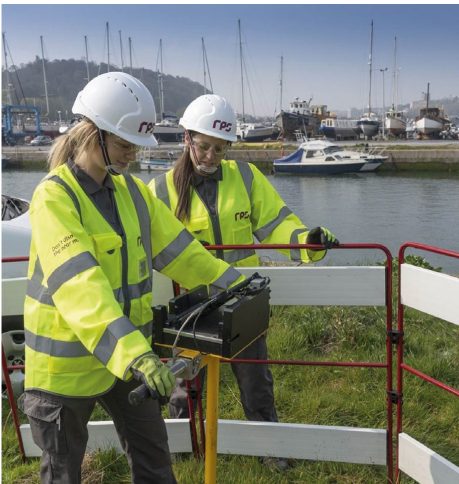
New technology is already helping to tackle leakage.
